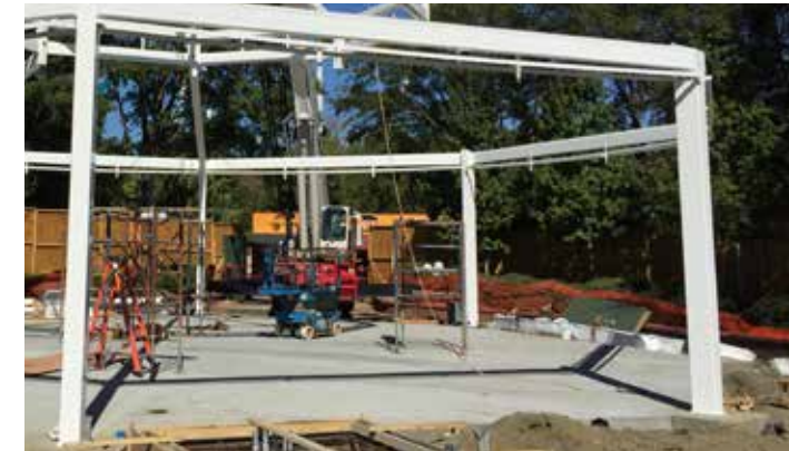
Frames are easily bolted together with provided fasteners
