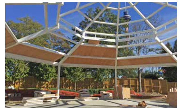
Supporting roof deck is installed
