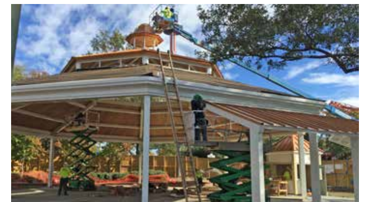
Installation of metal roofing panels
