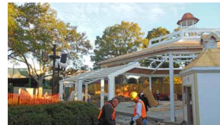
Installation of metal roofing panels
