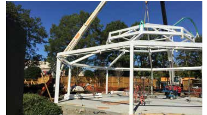
No field welding required during erection
